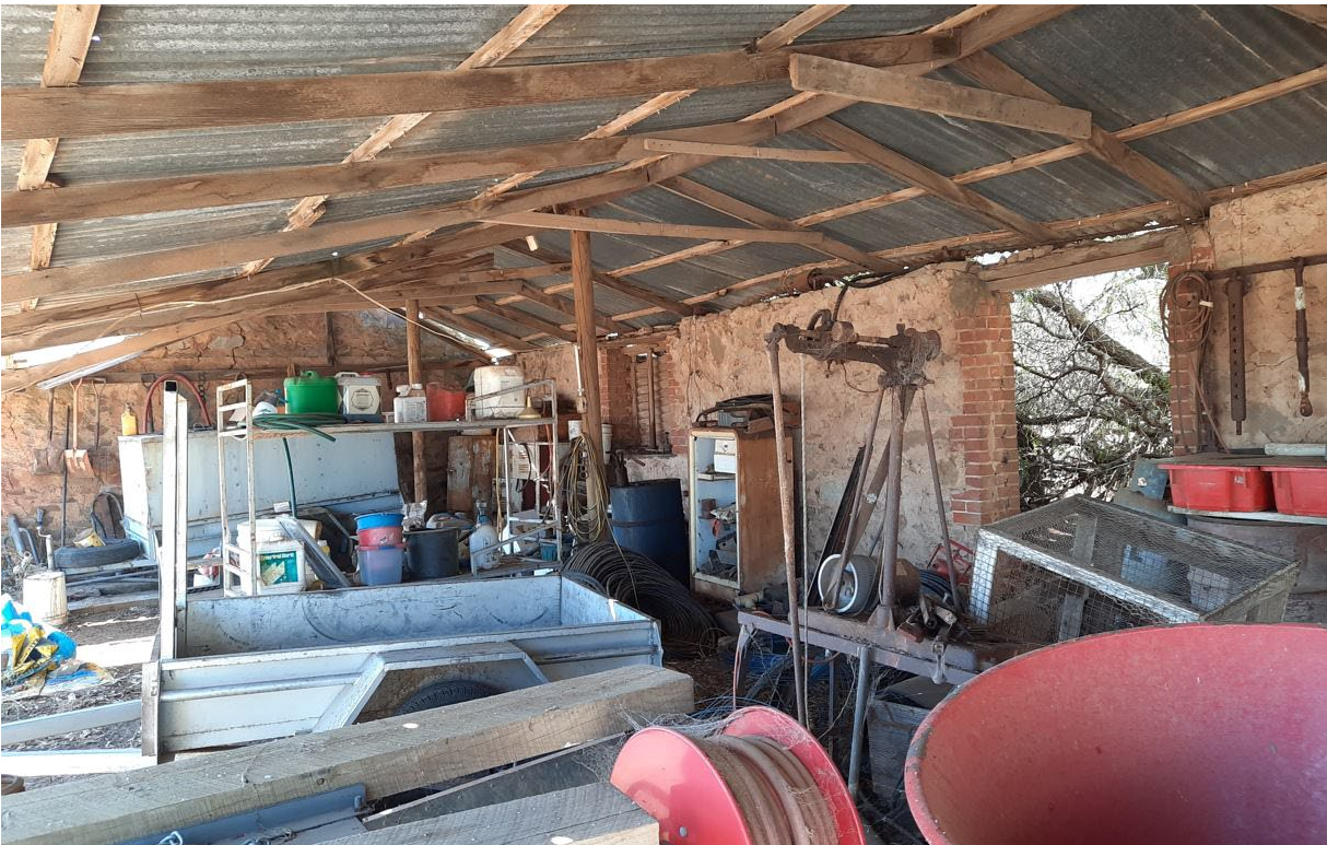
Later internal timber structure and corrugated steel roofing to outbuilding following removal of second storey, date unknown. (GGA, 2022).
