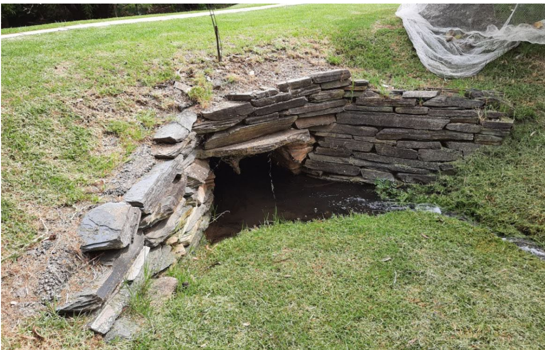
C.1840s slate culvert to former Government Quarry site, looking north (GGA, 2022)
