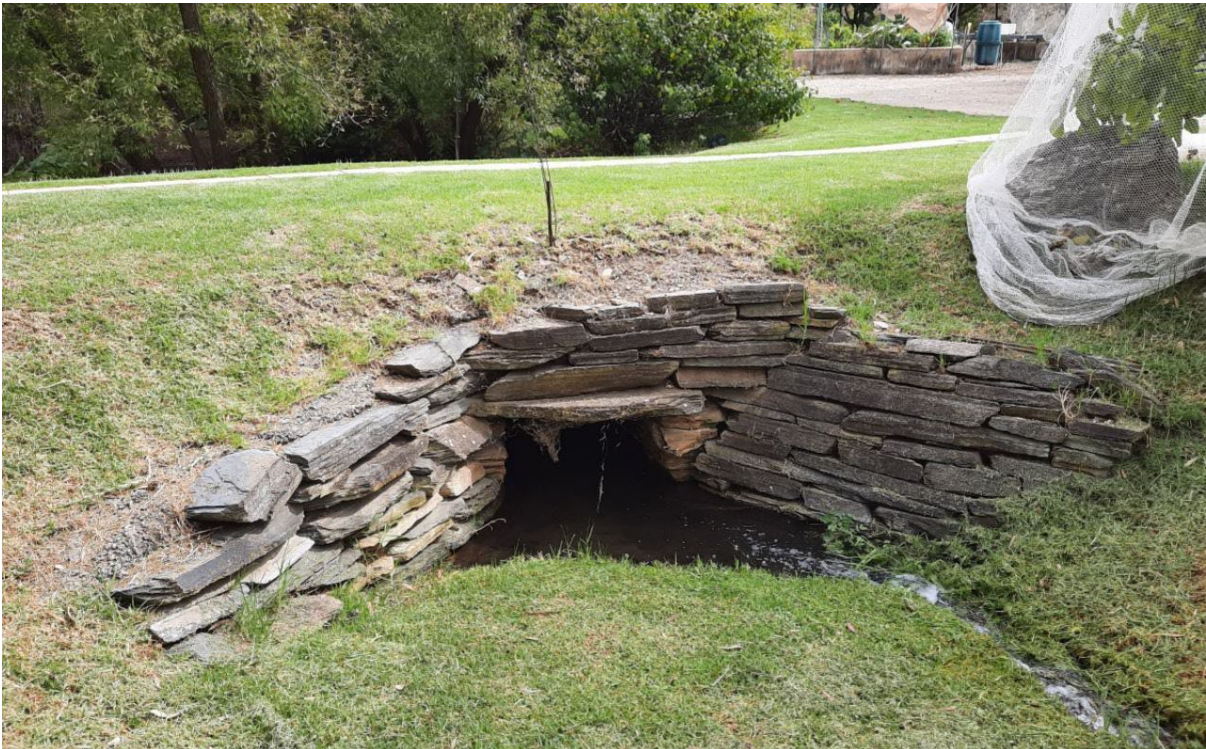
Slate culvert, 27 St James Street, Willunga (GGA, 2021)
