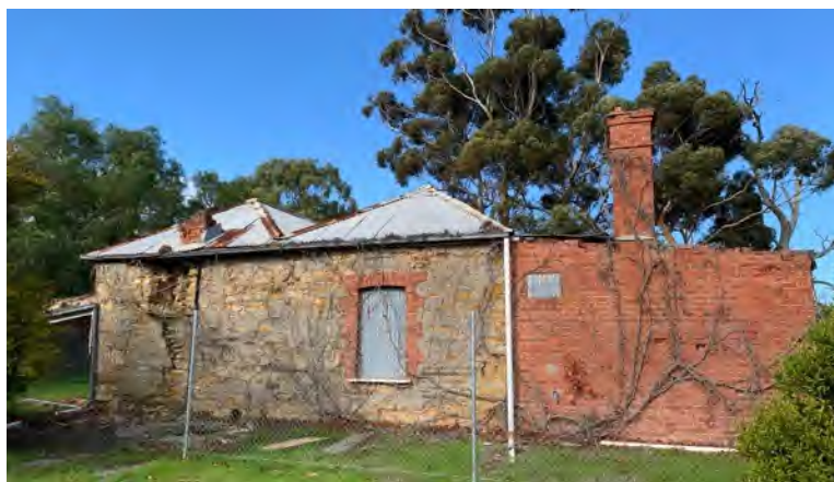
Figure 14: View from North Source: Anaglypta Architecture, 14 June 2022
