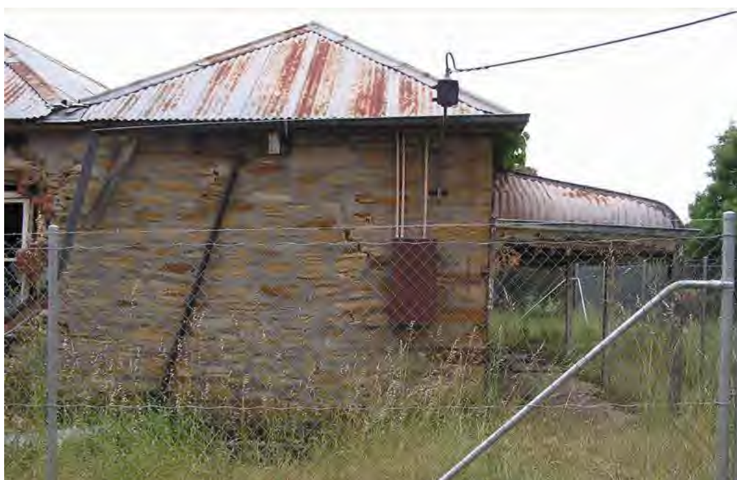
South elevation of former 'Rowlands' farmhouse (Andrew Stevens photographer).
