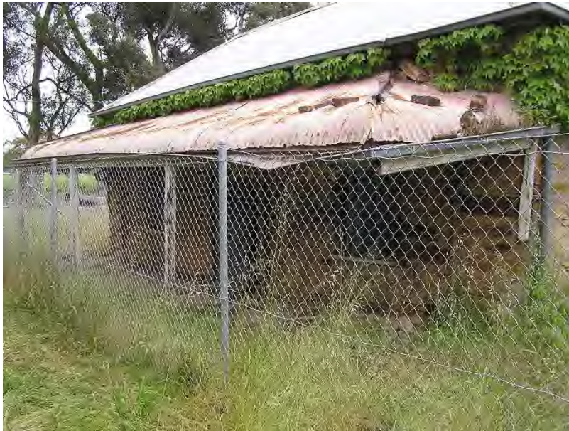
Photograph 2: The front verandah of the former farmhouse.
