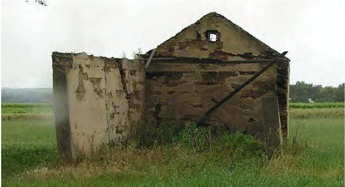
South elevation of Outbuilding No.1, looking north (Andrew Stevens, photographer).
