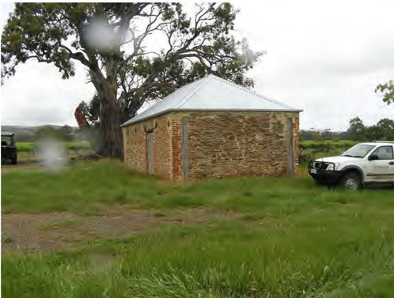
Photograph 10: Later, recently restored barn.
