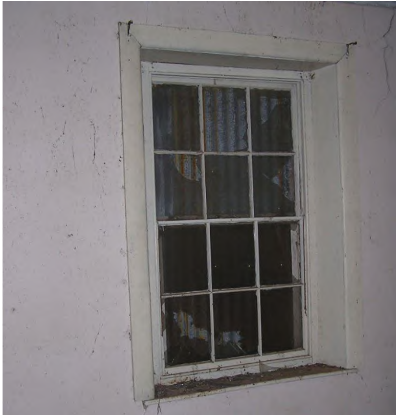
Victorian Regency styled window treatment to east façade windows, now covered in corrugated steel (Andrew Stevens, photographer).
