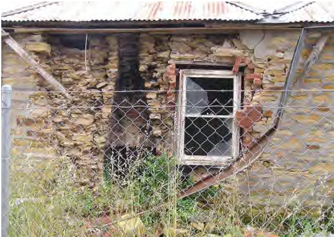
South elevation of former 'Rowlands' farmhouse, timber window with brick surrounds likely a later addition after the initial c.1853 construction (Andrew Stevens photographer).
