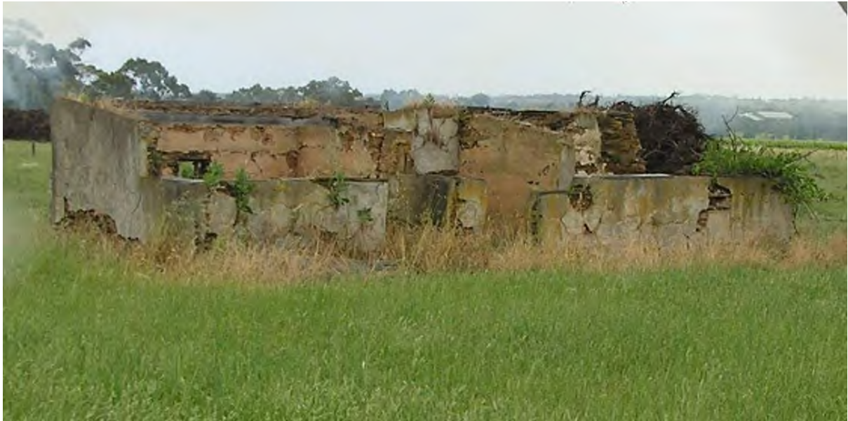
East elevation of Outbuilding No.2, looking west (Andrew Stevens, photographer).
