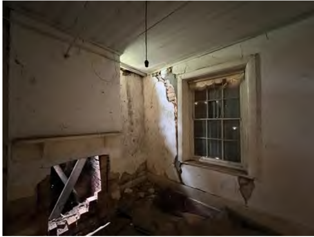
Figure 23: North East (Front) Room Source: Anaglypta Architecture, 28 January 2022
