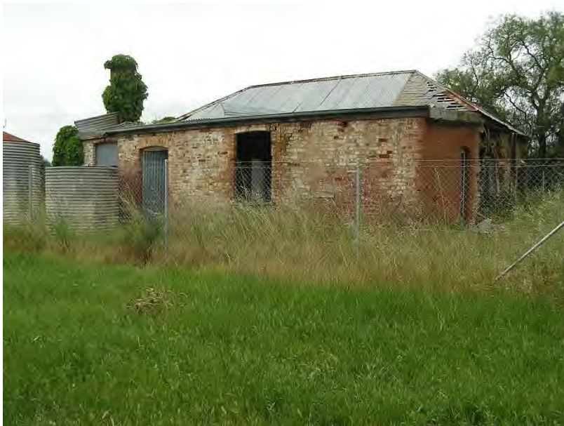
Photograph 4: The rear of the former farmhouse.
