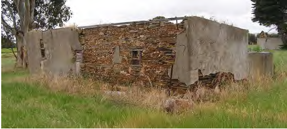
Outbuilding No.2, located south-west of the former farmhouse (Andrew Stevens, photographer)
