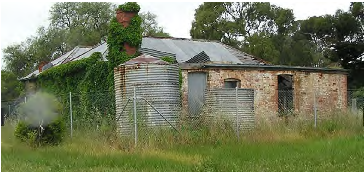
North elevation of former 'Rowlands' farmhouse covered in foliage, also showing early 20 th century rear lean-to additions and 20 th century rainwater tanks (Andrew Stevens photographer).
