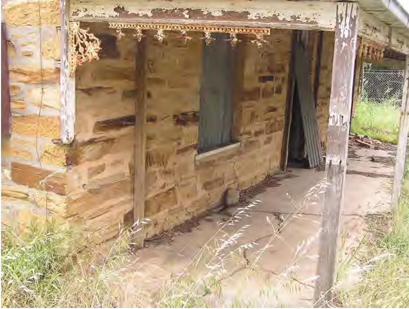
Photograph 5: The front wall of the former farmhouse.
