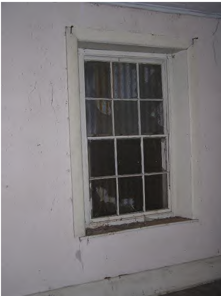
Photograph 6: Multi-paned front window of the former farmhouse.
