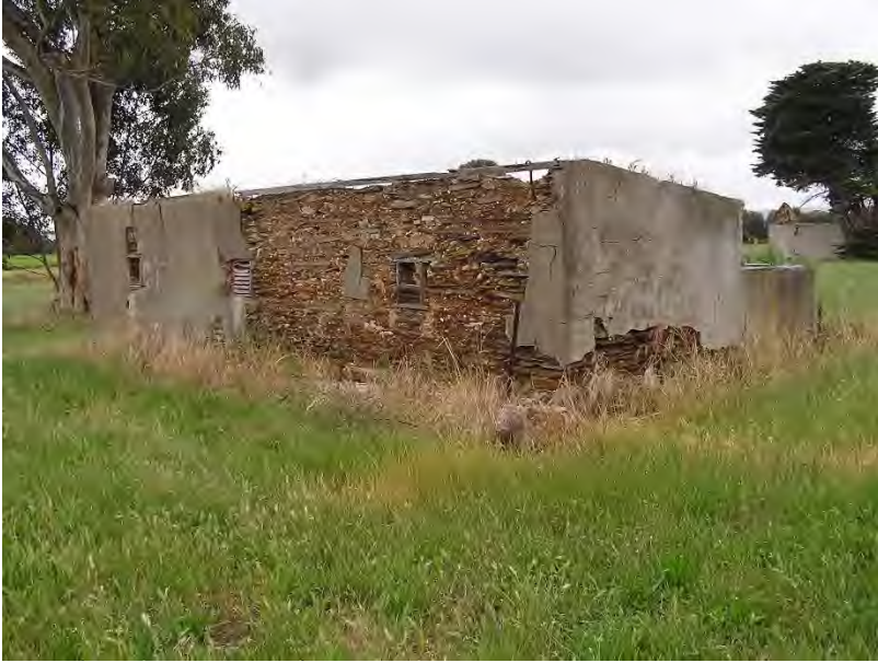
Photograph 9: Outbuilding, likely former animal enclosure building.
