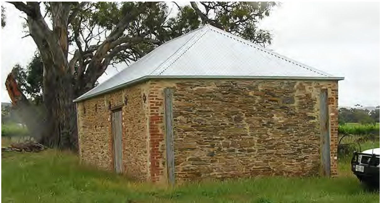
East elevation of Outbuilding No.3, looking west (Andrew Stevens, photographer).
