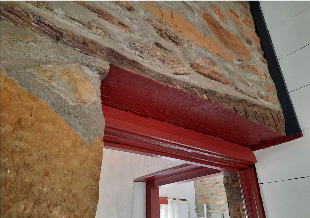
Early rough-hewn timber lintel to door between kitchen and living room (GGA, 2022)
