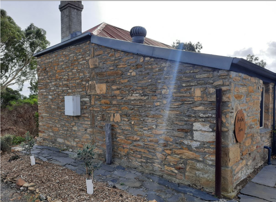
Early fabric relating to the west elevation of the c.1850s residence (GGA, 2022)
