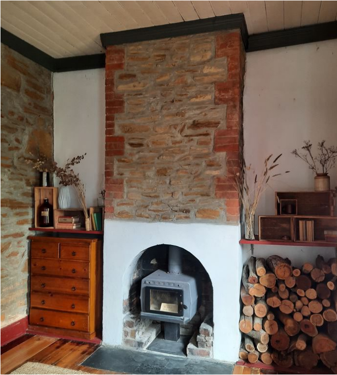
Exposed stonework with brick quoins to living room fireplace, likely dating to the late 19 th century (GGA, 2022).
