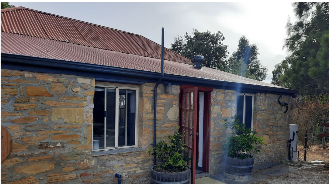
South elevation of c.1850s residence, showing later aluminium windows and timber and glass door to early lean-to openings (GGA, 2022)
