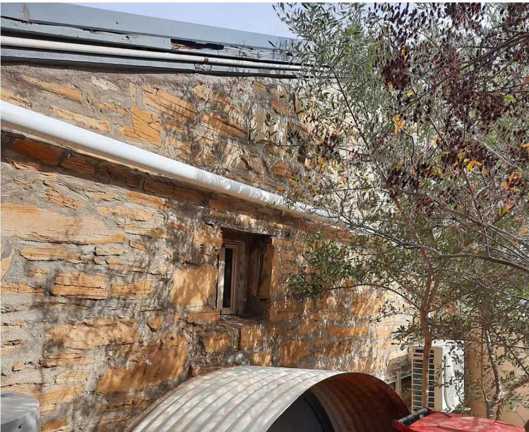
Early fabric of the east elevation of the c.1850s residence, with later timber eaves elements (GGA, 2022)
