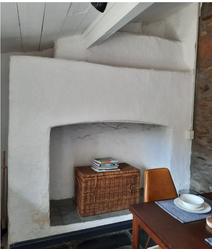
Early masonry fireplace to lean-to kitchen (GGA, 2022)
