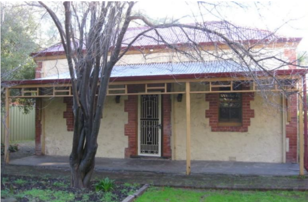
West elevation of 413b Main Road, Coromandel Valley ( https://www.realestate.com.au/property/413b-main-rd-coromandel-valley-sa-5051 , accessed 18/1/2022).
