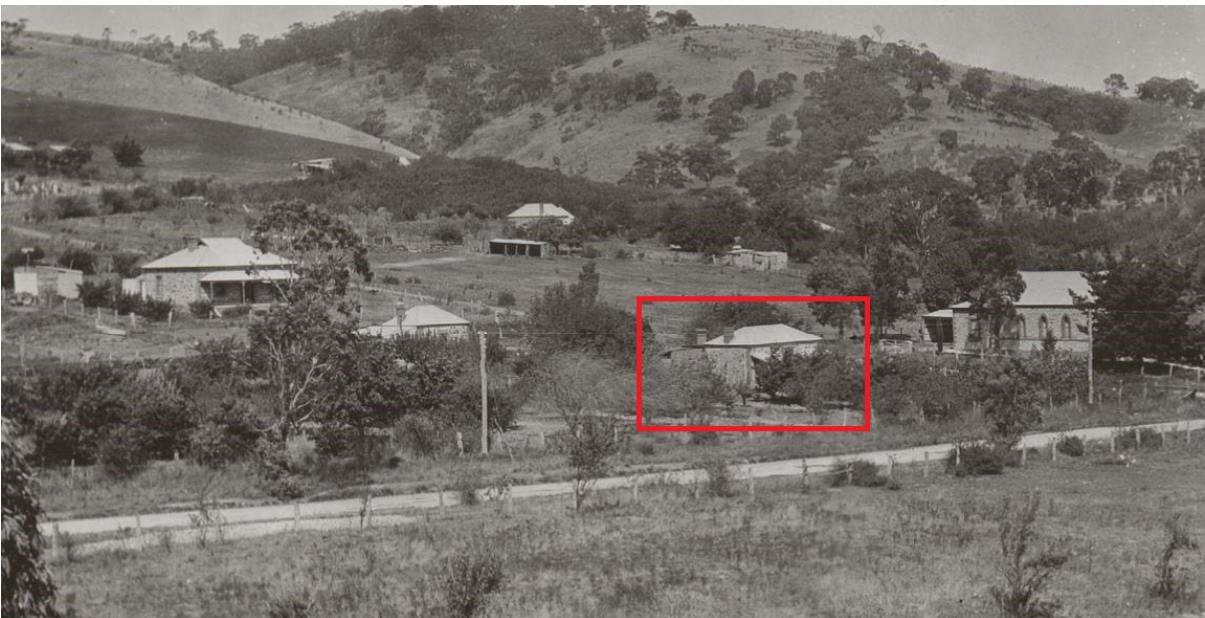
C.1912 photograph of 413b Main Road, Coromandel Valley, highlighted within red box (SLSA B 28529)
