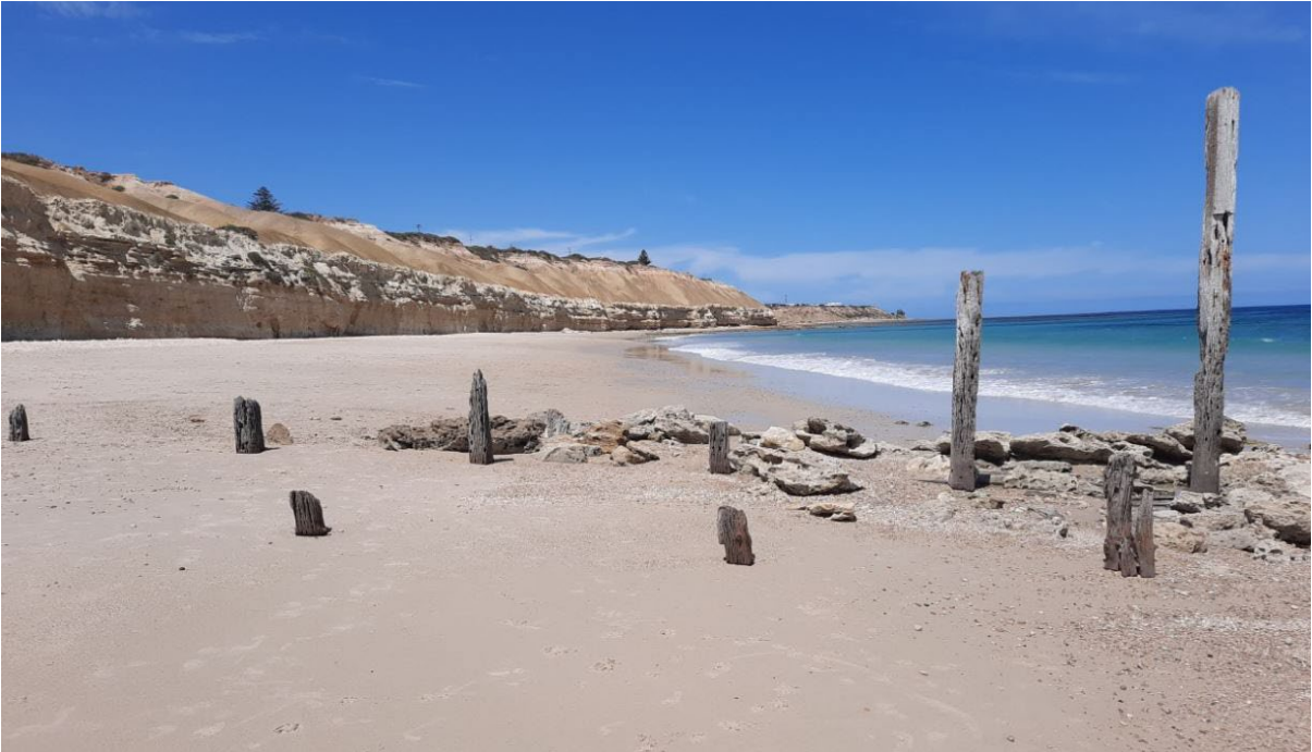
Timber remnants of the c.1868 timber retaining walls of the former jetty embankment, looking south (GGA, 2022)
