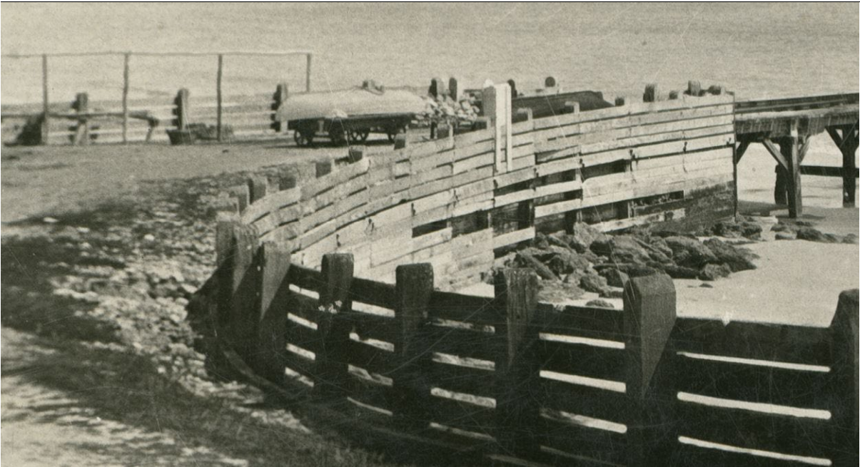
Pre-1915 photograph of north-side of Port Willunga jetty embankment, with timber retaining wall infrastructure and footing, now the remaining fabric of the Port Willunga jetty pylons (SLSA, B 7451).
