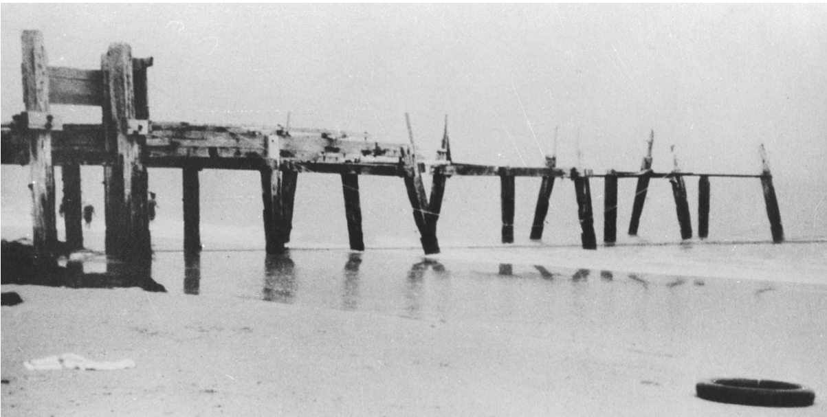
C.1930 photograph of Port Willunga Jetty ruins (SLSA, B 55417/263)
