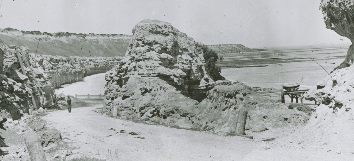
C.1910 photograph of ramp approaching Port Willunga Jetty, embankment infrastructure can be seen to the right of image (SLSA, B 13320)
