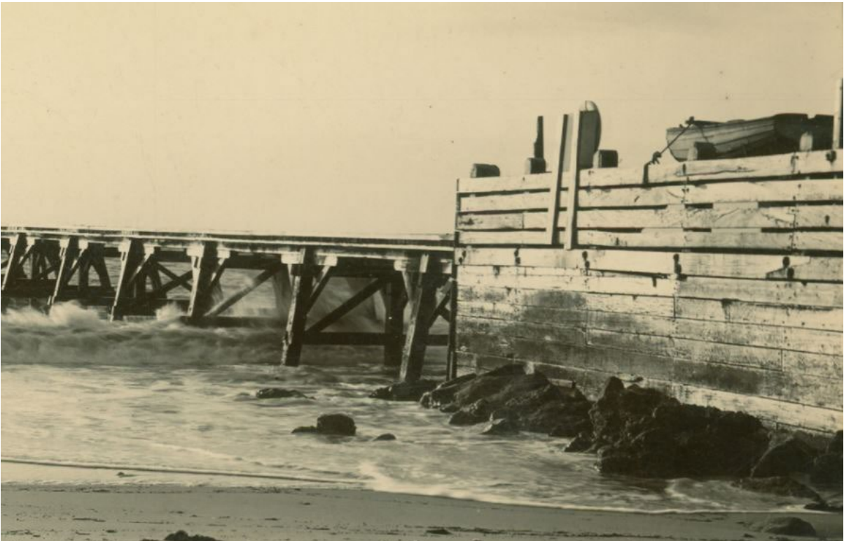
C.1905 photograph of south-side Port Willunga jetty embankment, with timber retaining wall infrastructure and footing, now the remaining fabric of the Port Willunga jetty pylons (SLSA, B 22137).
