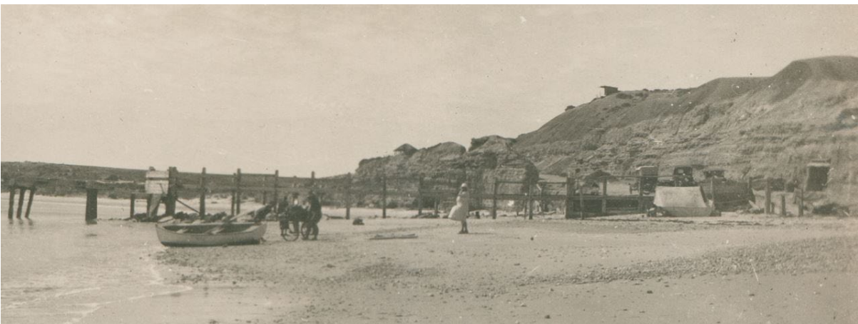
Port Willunga jetty site in the c.1920s (SLSA description erroneously attributes a date of c.1910), showing reconfigured 'boardwalk' construction to the jetty remnants after the destructive 1915 storms (SLSA, B 16429)
