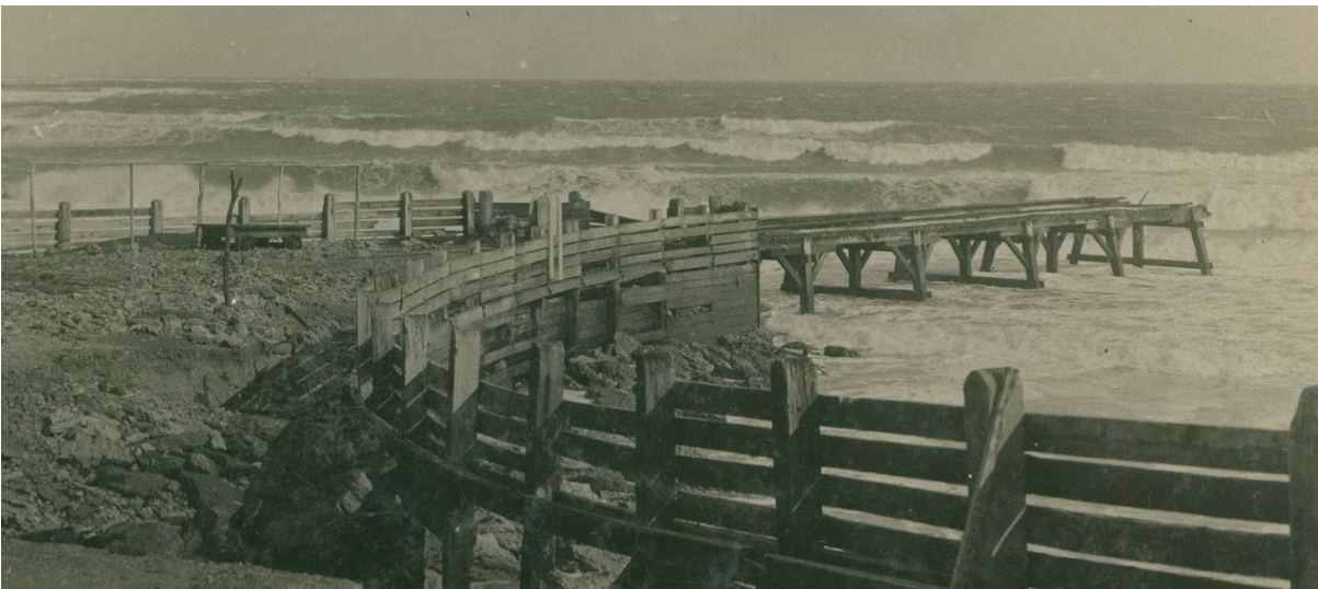
Remains of Port Willunga Jetty and associated embankment after storms in 1915 (SLSA, B 11918).
