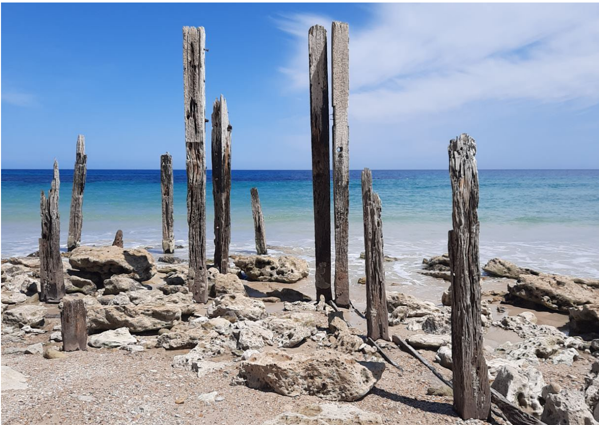
Timber remnants and stone foundations of the Port Willunga Jetty embankment and subsequent 'boardwalk', looking west. Later vertical timbers are understood to relate to the post-1915 'boardwalk', with deteriorated timbers relating to the c.1868 timber retaining walls of the former jetty embankment (GGA, 2022)
