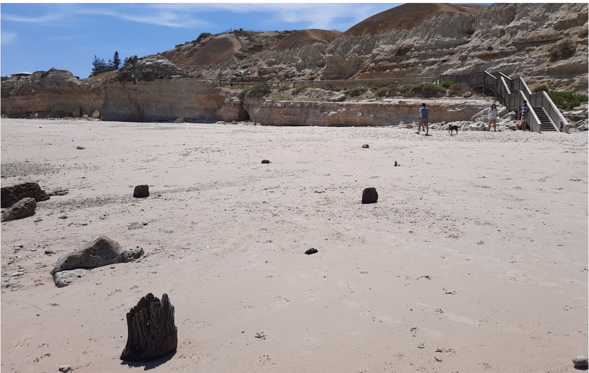
Timber remnants of the c.1868 timber retaining walls of the former jetty embankment extending east to the c.1868 ramp, looking east (GGA, 2022)
