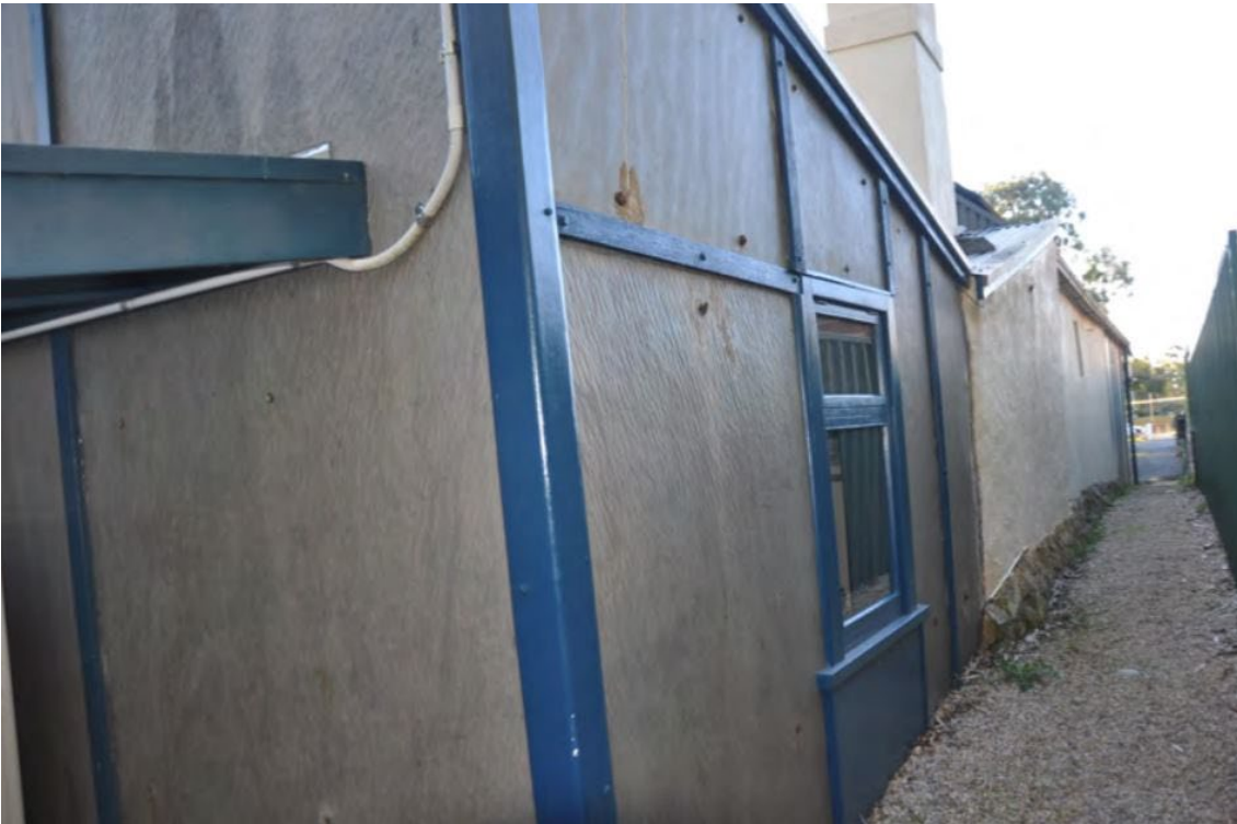
External slate fabric to rear c.1920s additions at 24 Peters Terrace, Willunga, looking north; fabric to the east elevation appears to be largely in original condition. (National Trust of South Australia, Willunga Branch).
