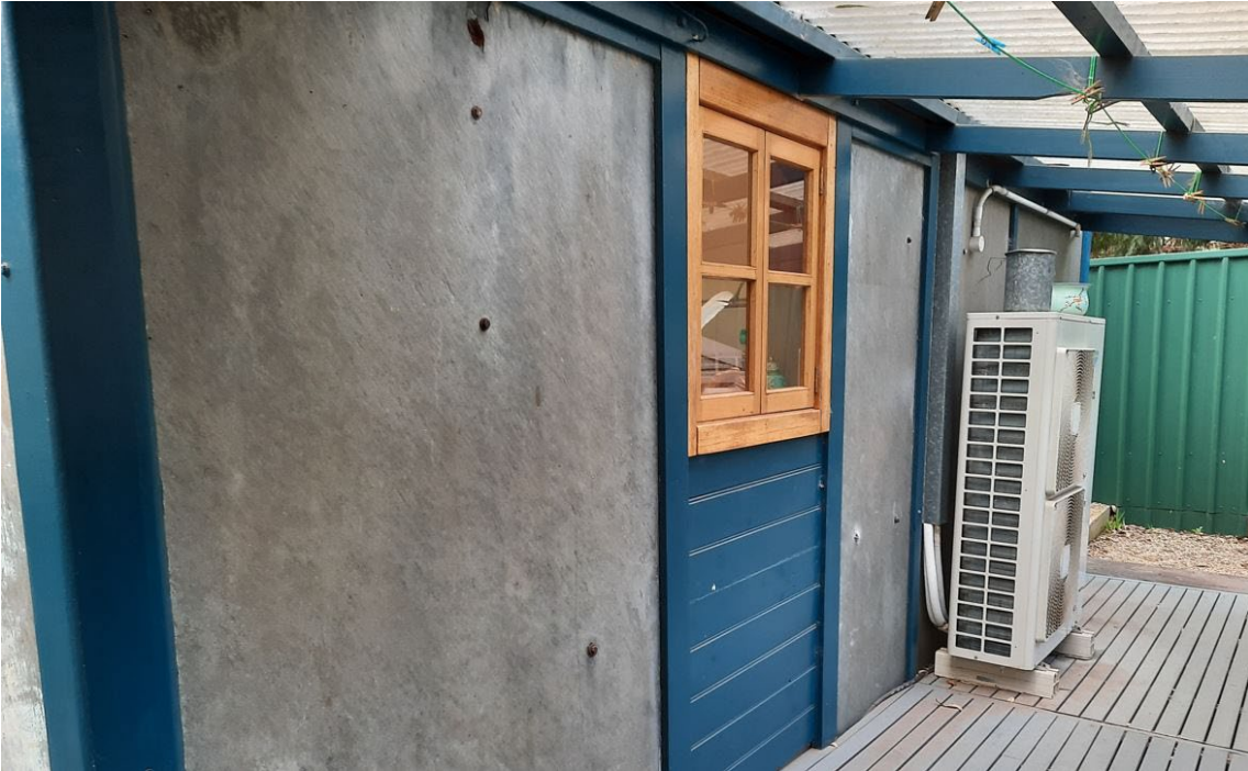
External slate fabric to rear c.1920s additions at 24 Peters Terrace, Willunga, looking east. Note later additions including external air conditioning, piping and later timber window are not recommended for inclusion in the extent of listing (GGA, 2022)
