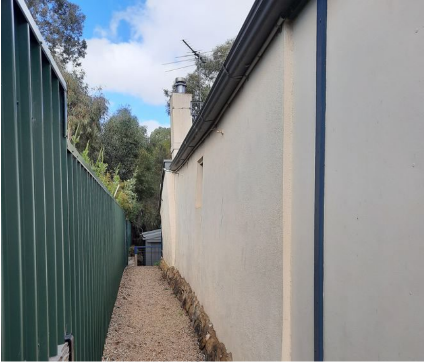
C.1850s pug construction to east elevation of residence, with later external concrete rendering. (GGA, 2022)
