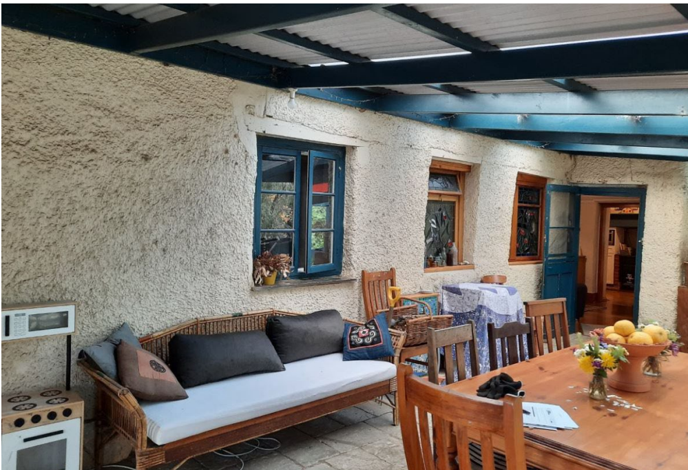
C.1850s pug construction to west elevation of residence, with later external concrete rendering. Early window form with casement window and inscribed slate sill, extensive alterations to other early window and door forms to this elevation. Late 20 th century verandah extending to the west from elevation. (GGA, 2022)
