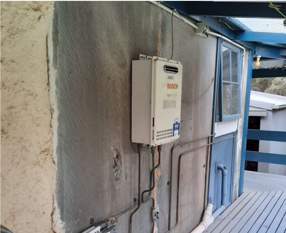
External slate fabric to rear c.1920s additions at 24 Peters Terrace, Willunga, looking south-east. Note later additions including external water heater, piping and fibreboard infill are not recommended for inclusion in the extent of listing (GGA, 2022)
