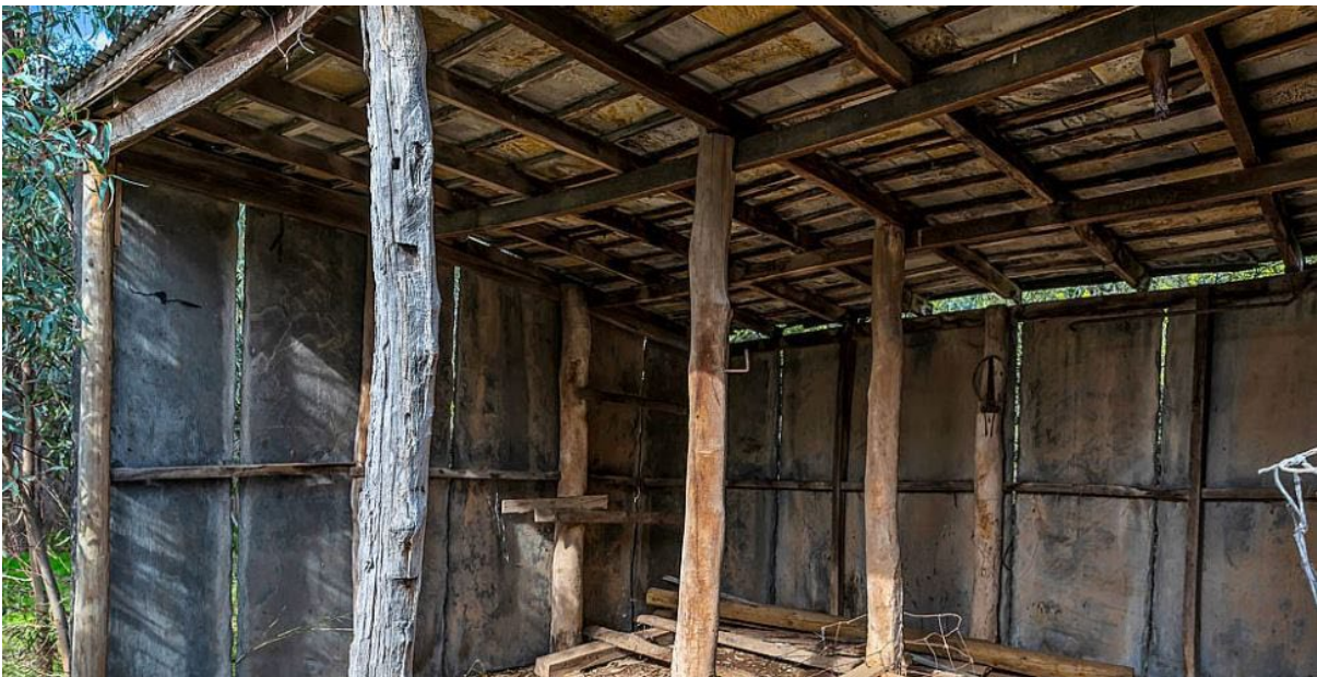
Internal timberwork and slate external fabric of slate stables at 7 St Lukes Street, Willunga, looking north ( https://www.realestate.com.au/property/7-st-lukes-st-willunga-sa-5172 , accessed 20/4/2022).
