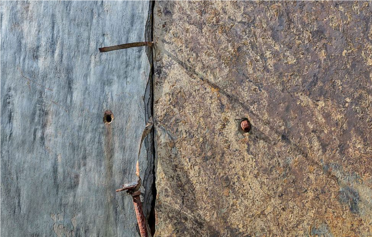
External slate cladding with early metal ties and rods at 7 St Lukes Street, Willunga, looking east ( https://www.realestate.com.au/property/7-st-lukes-st-willunga-sa-5172 , accessed 20/4/2022).
