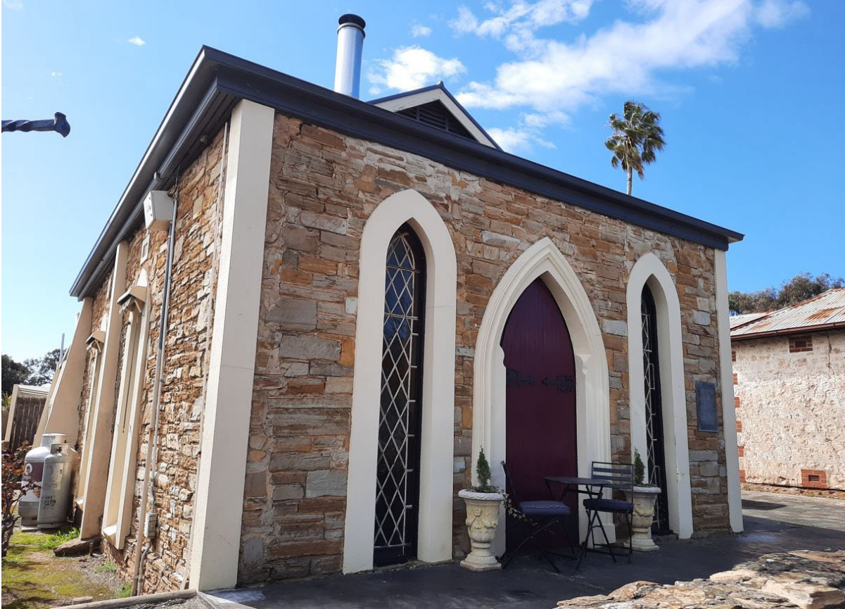
Former Primitive Methodist Chapel, 27 High Street, Willunga (GGA, 2021)
