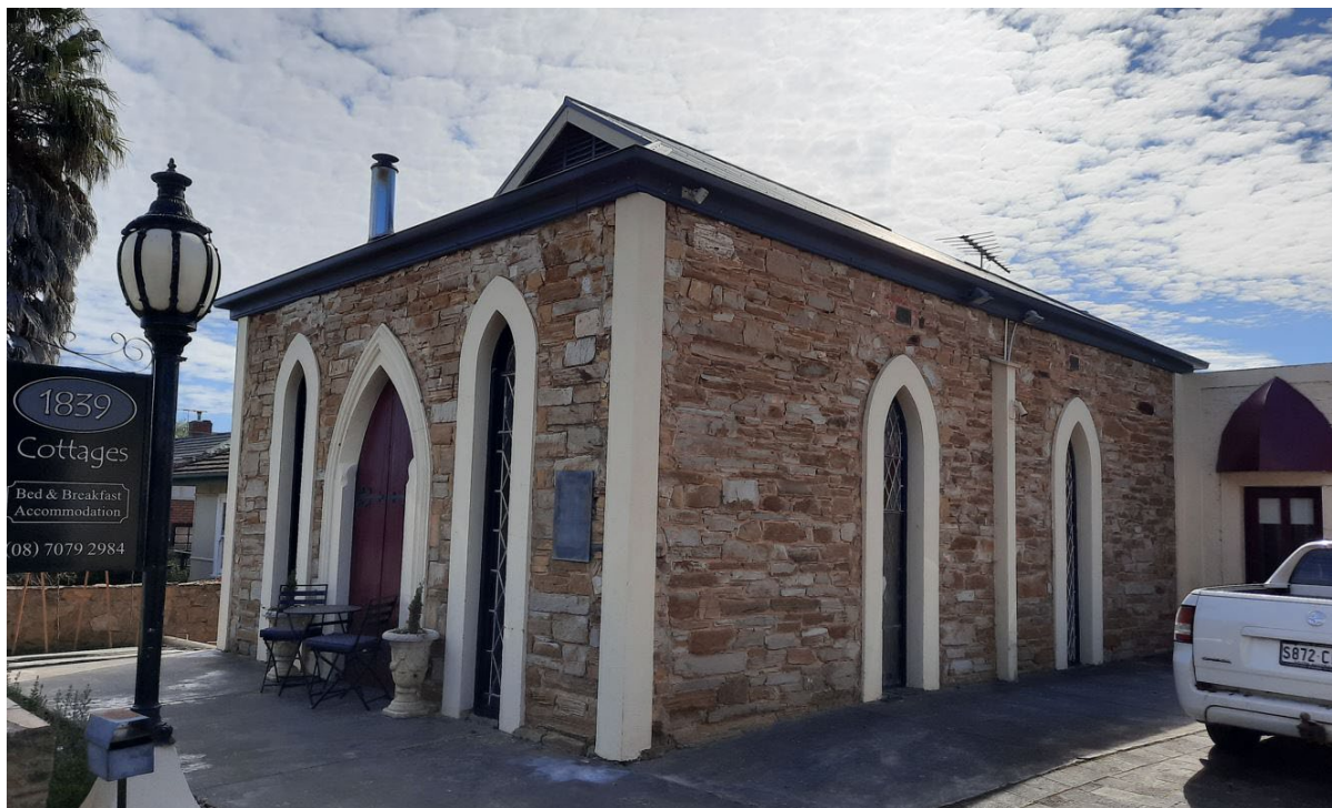
Former Primitive Methodist Chapel, 27 High Street, Willunga (GGA, 2021)
