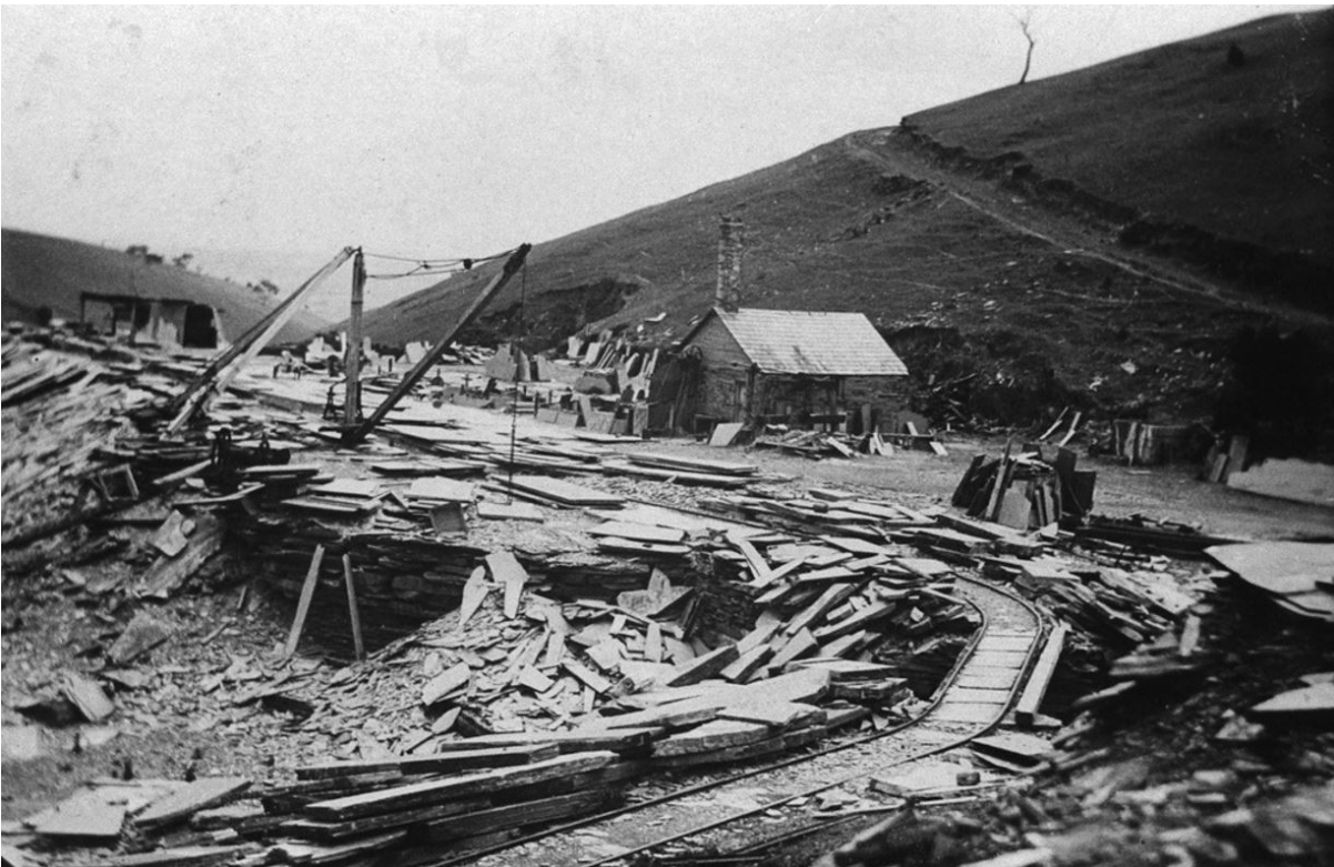
C.1908 photograph of Martin's Slate Quarry in Beltana (Beltunga?) Gully (SLSA, B 55417/90)
