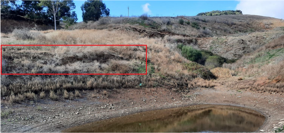
Site of quarry pool; retaining wall located to eastern embankment (shown within red box), looking east (GGA, 2022).
