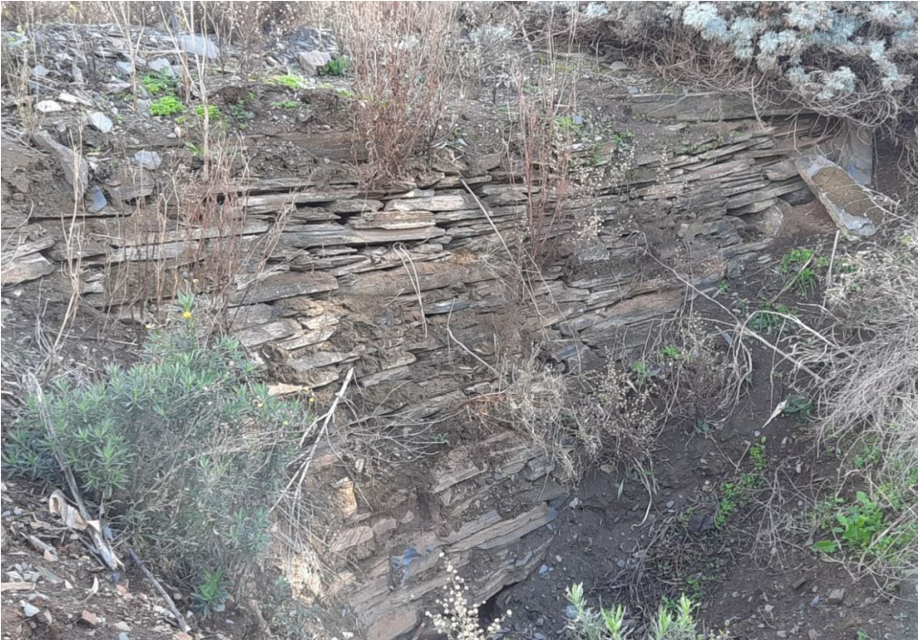
Slate fabric to right-hand side of culvert, located immediately south of the quarry entrance from Quarry Road, looking west (GGA, 2022).
