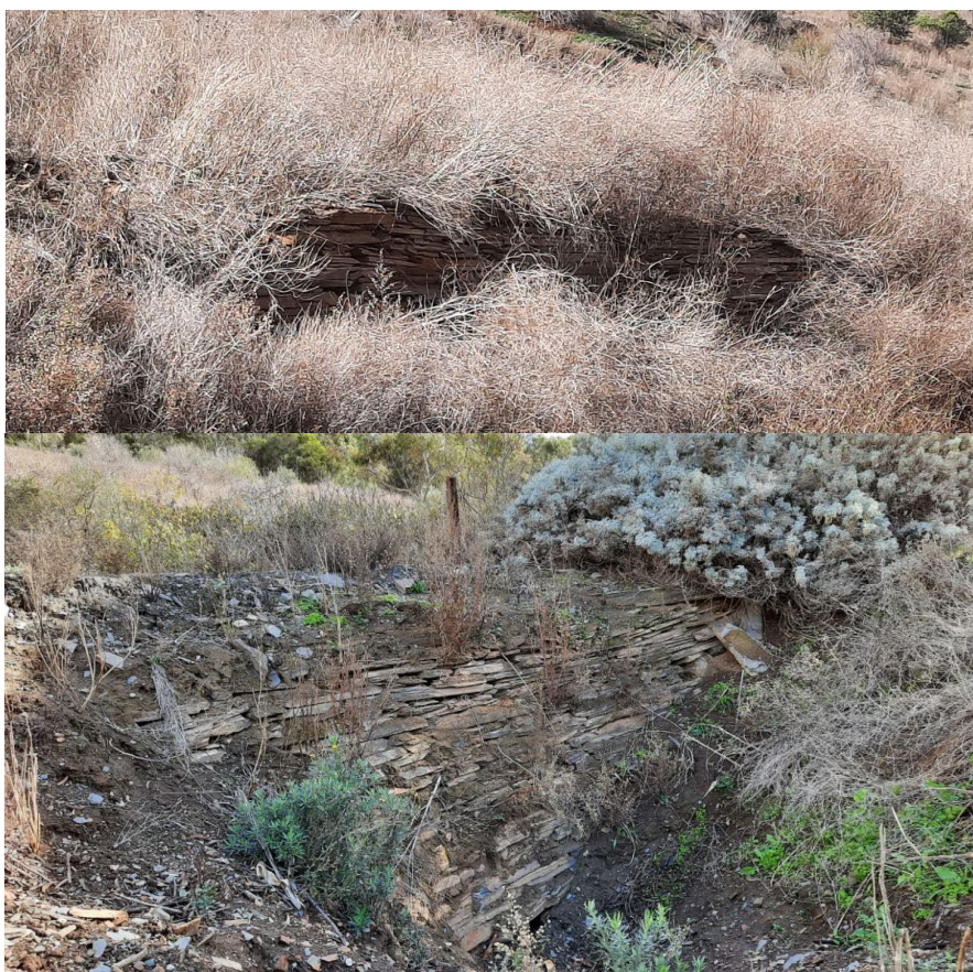
Slate retaining wall and culvert to Martin's & Bastian's Quarry, 81 Quarry Road, Willunga South (GGA, 2022).
