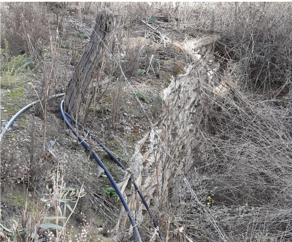
Slate fabric to left-hand side of culvert, located immediately south of the quarry entrance from Quarry Road, looking south-west (GGA, 2022).
