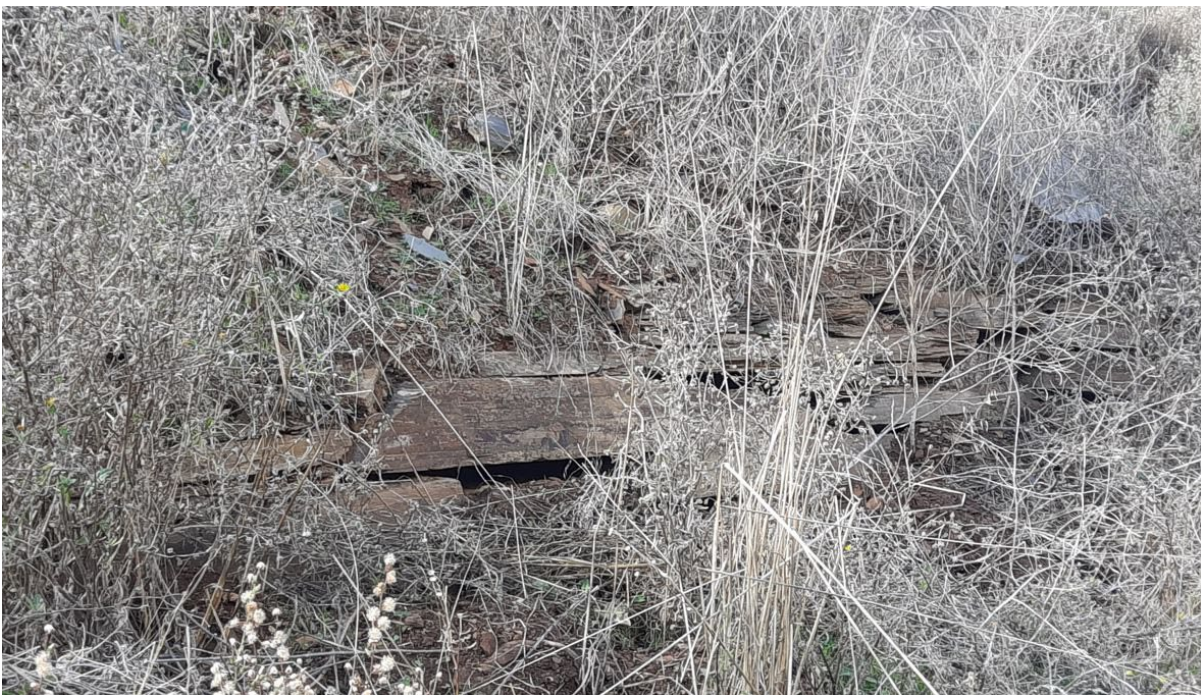
Additional partially-buried slate fabric to slate retaining wall, looking east (GGA, 2022).
