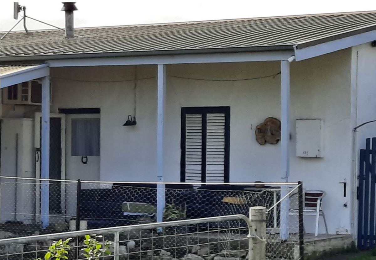
French doors and shutters, believed to date to original construction (c.1870s), little other surviving heritage fabric (GGA, 2021).
