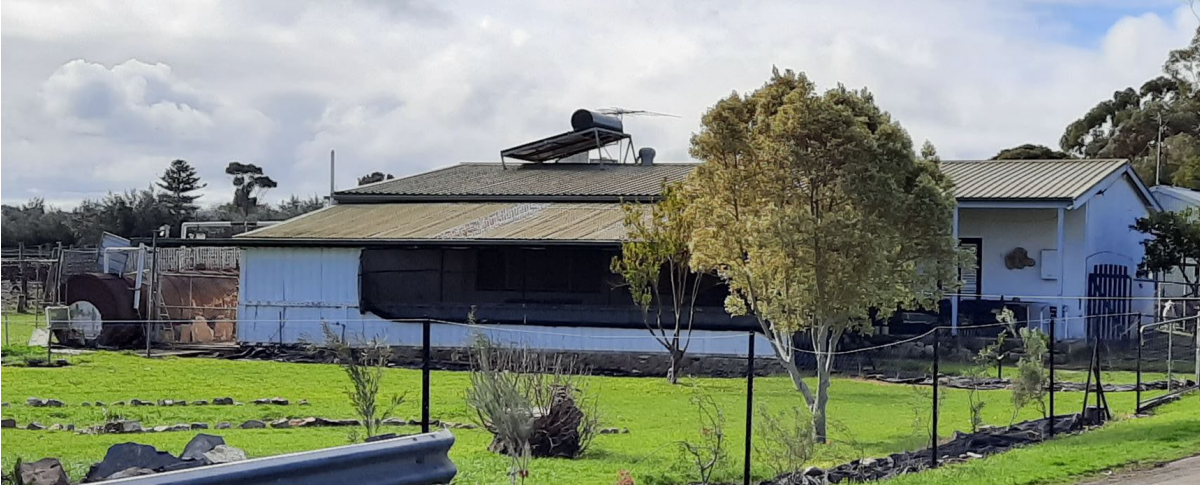
Extensive additions and modifications to 94 Flour Mill Road, Whites Valley (GGA, 2021).
